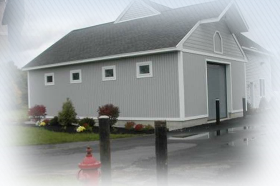
Manganese Removal Facility
